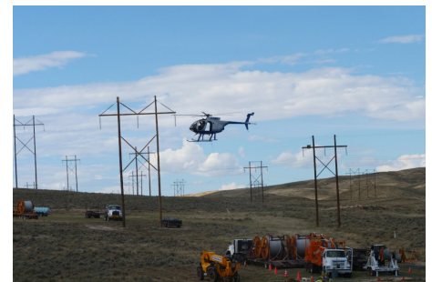
Ready Wyoming construction activity
