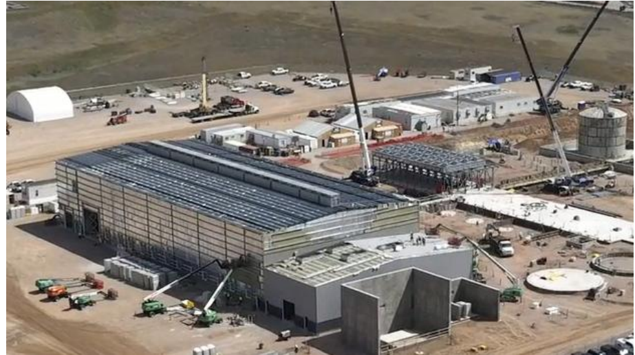
Pictured: Lange II generation project site under construction in Rapid City, South Dakota
