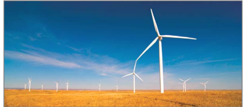
Pictured: Happy Jack Wind Farm located near Cheyenne, Wyoming, serves Wyoming and South Dakota Electric (owned by Duke Energy)
