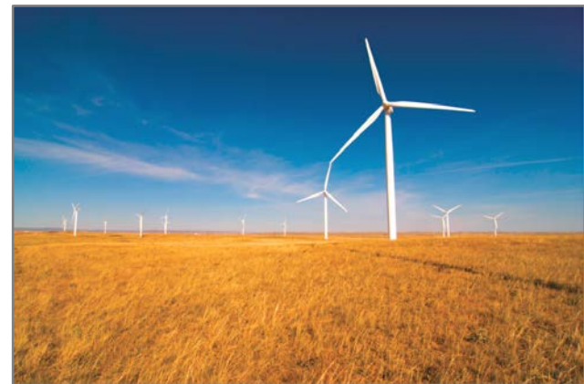
Pictured: Happy Jack Wind Farm located near Cheyenne, Wyoming, serves Wyoming and South Dakota Electric (owned by Duke Energy)
