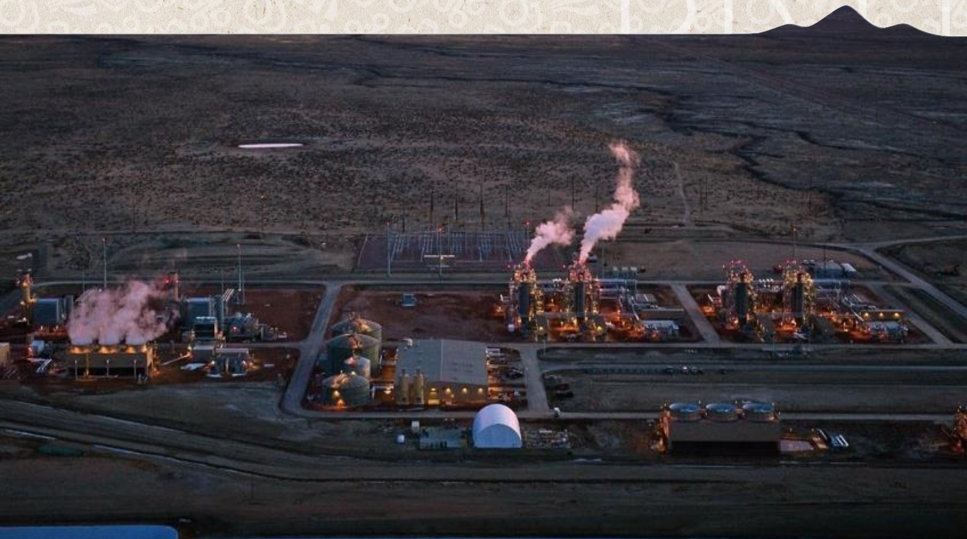
Pueblo Airport Generating Station near Pueblo, Colorado
