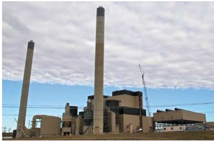
Figure 05-6. Wygen II and Wygen III Generation Facility
