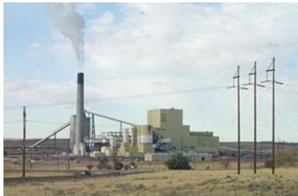
Figure 05-7. Wyodak Generation Facility
