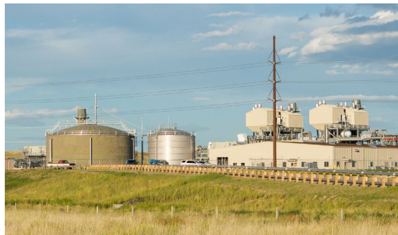
Figure 05-8. Cheyenne Prairie Generating Station Combined Cycle CT
