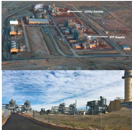
Pueblo Airport Generating Station
