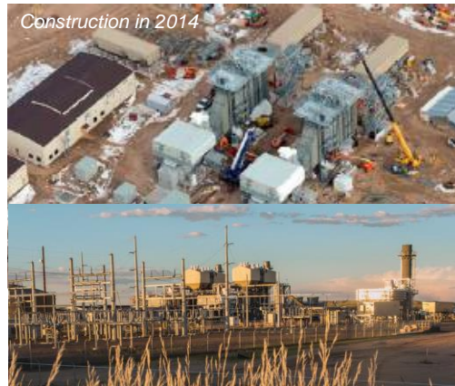
Cheyenne Prairie Generating Station
