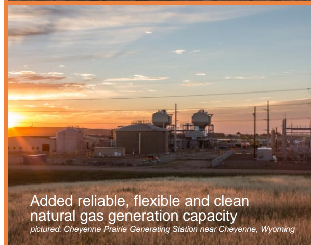
Responsibly adding renewable resources pictured: Busch Ranch II wind project in Pueblo, Colorado
